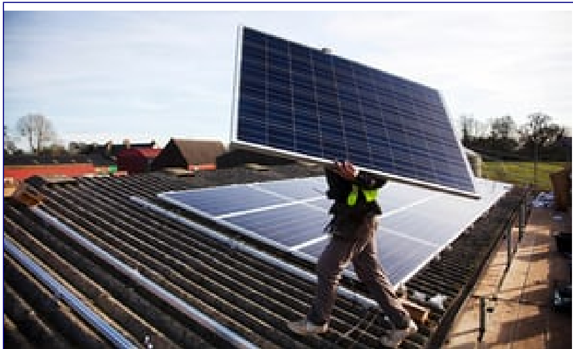
Solar panel installation. Photograph: Kristian Buus/Corbis via Getty Images
