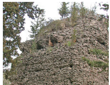
Example of opus caementicium on a tomb on the ancient Appian Way in Rome. The original covering has been removed.
