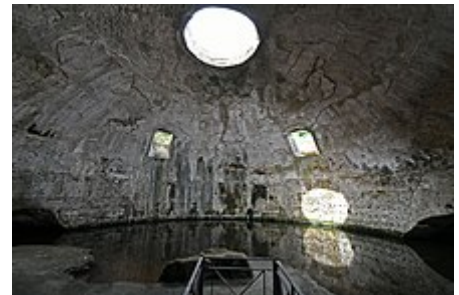
Ruins of the so-called "Temple of Mercury" in Baiae , a Roman frigidarium pool of a bathhouse built in the 1st century BC during the late Roman Republic, [6] containing the oldest surviving concrete dome , [7] and largest one before the Pantheon . [8]
